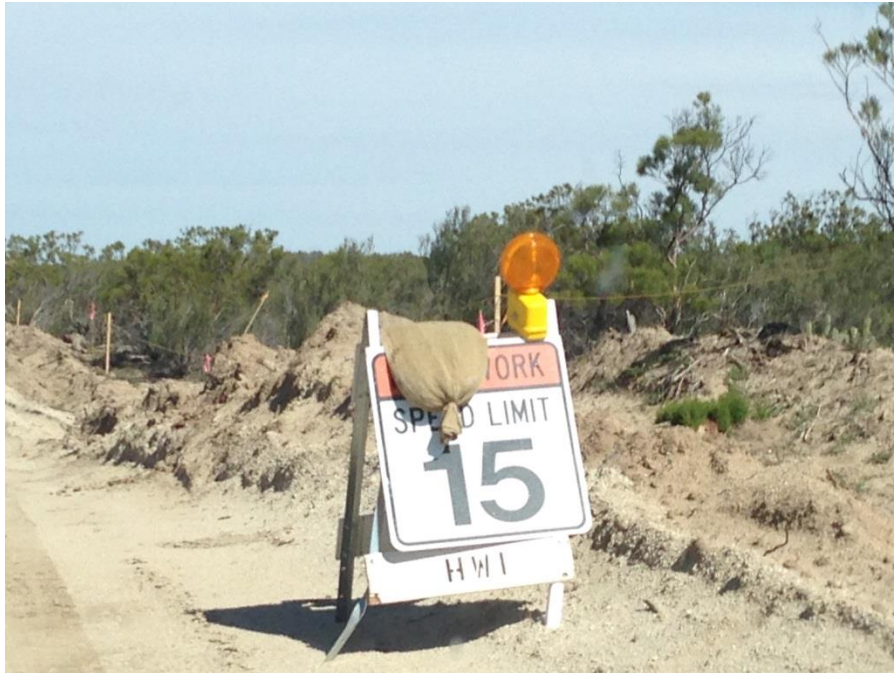
Photo 6: In accordance with MM-BIO-7b, speed limit signage has been placed along access roads to enforce speed limits in and around all construction areas.
