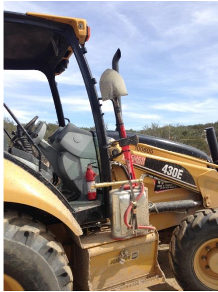
Photo 5: In accordance with MM-FF-1 and the Construction Fire Prevention/Protection Plan, fire equipment was observed to be present on construction equipment.
